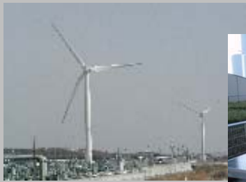
wind generators in the waterfront area
